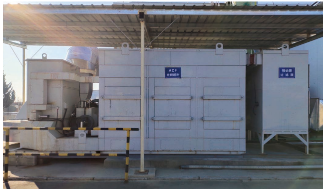
Organic Waste Gas Catalytic Combustion Purification Device 有機廢氣催化燃燒淨化裝置
